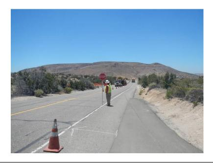
**Photo 4:** Traffic cones and flaggers present along Old Highway 80 in accordance with Mitigation Measure TRA-1.
