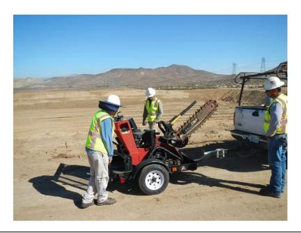
**Photo 5:** Construction equipment is inspected and verified to be clean and free from dirt and debris prior to being unloaded on-site to minimize the spread of invasive plant species in accordance with Mitigation Measure BIO-3a.
