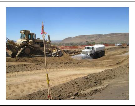
**Photo 1:** Water trucks are utilized during grading activities to minimize fugitive dust in accordance with Mitigation Measure BIO-4a and the Dust Control Plan.
