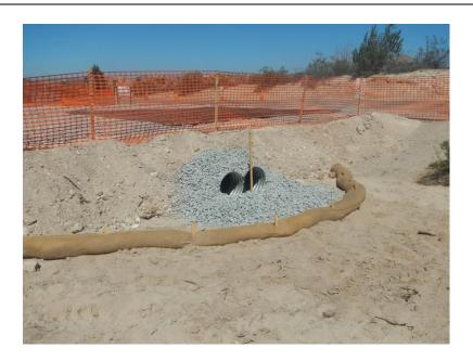
**Photo 2:** BMPs are installed along the right-of-way to minimize the potential for erosion in accordance with Mitigation Measure HYD-1 and the SWPPP.
